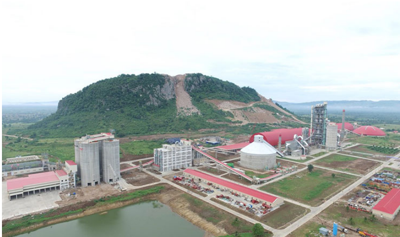
Battambang Conch Cement Factory is a joint venture of local and Chinese investors. AKP
